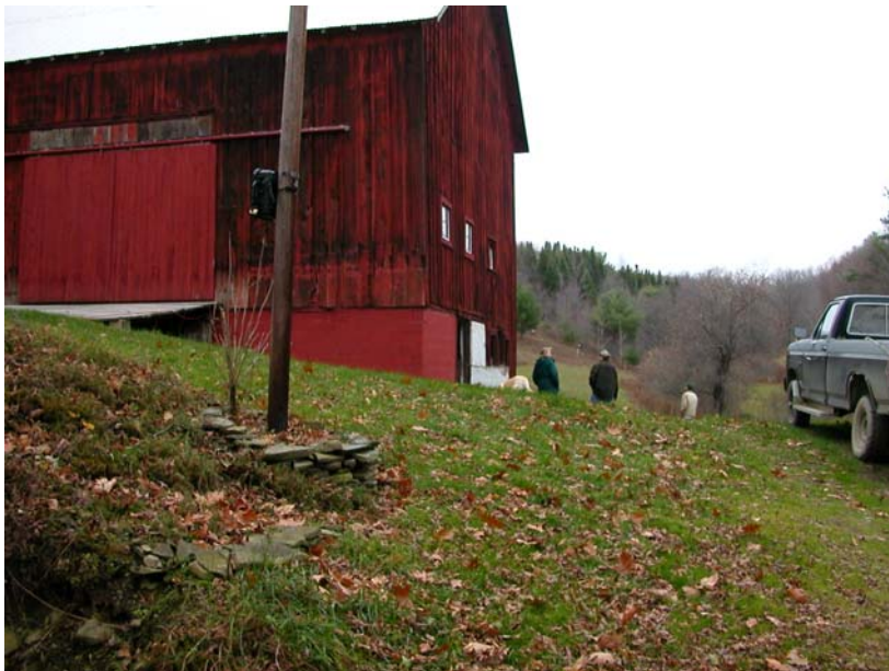
Figure 2.2.4 Main Site South Location – Looking N
