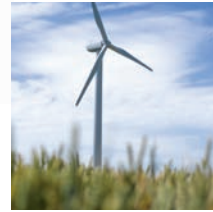
Haute Lys, France 25 x 1.5s total capacity: 37.5 MW
