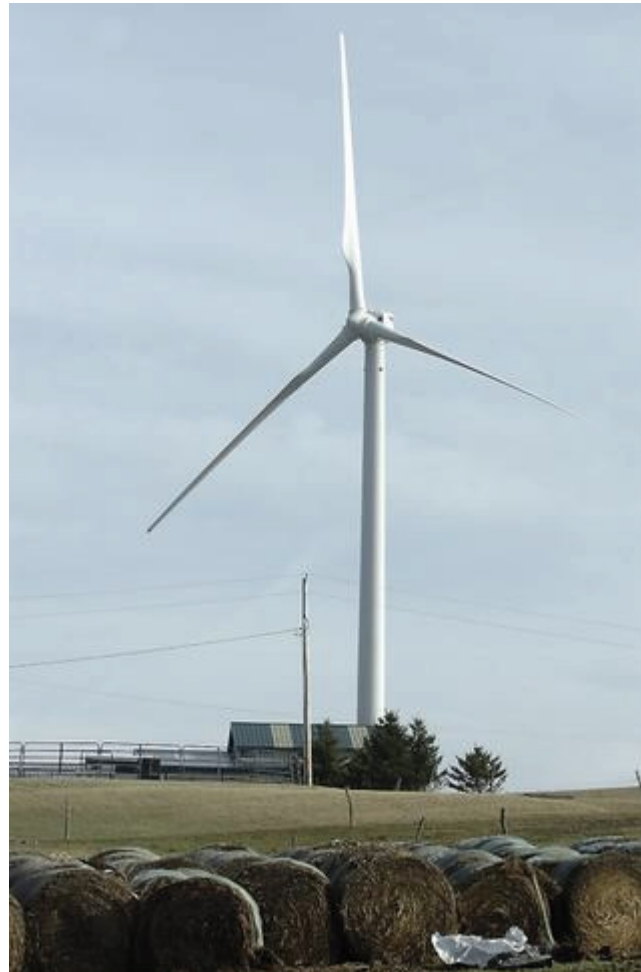
This wind mill is part of the Dutch Hill wind farm in Cohocton. Plans to open a wind farm in Prattsburgh have been put on hold, developer First Wind announced Monday.
