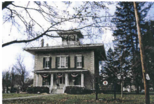
Larrowe House (Cohocton Municipal Building)
